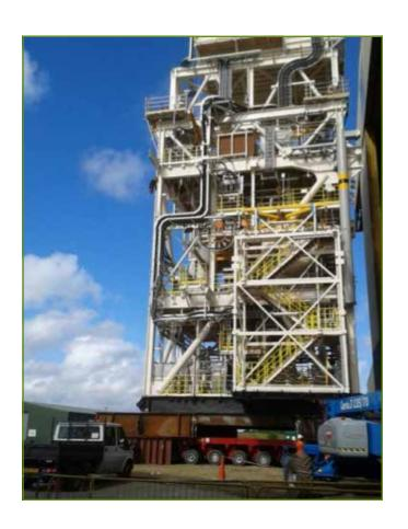
The newly fabricated module was to be "bolted on" to the existing platform, which required key weight considerations for the design. As well as the construction of the module itself, the project also encompassed the challenge of associated brownfield works necessary to "hook up" the module with the existing platform.
